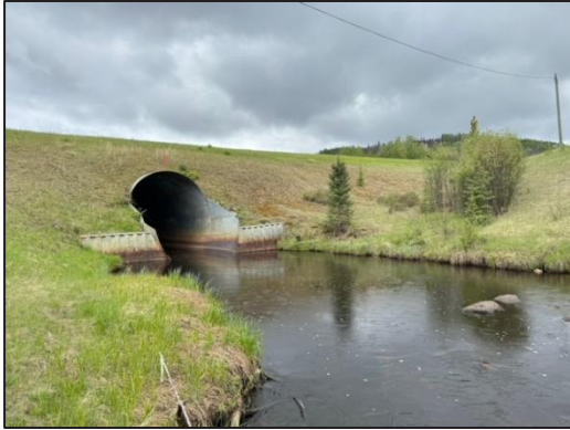
a. Highway culvert outlet and sensor gauge pool, June 14, 2024.
