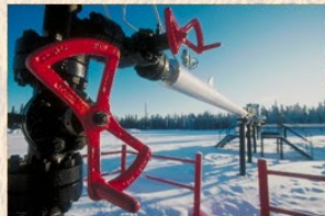
Engineering & Safety Research
